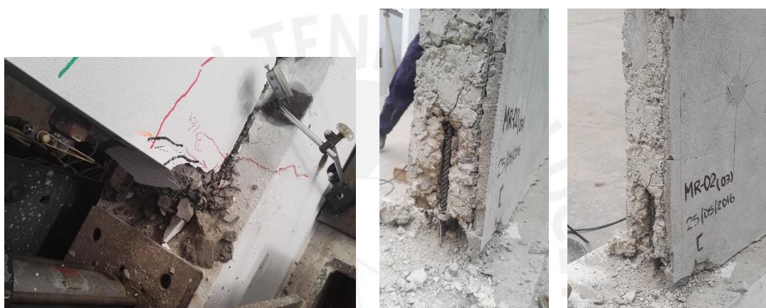
Figura 6.49. Estado final post-ensayo MDL02-R-SCA
